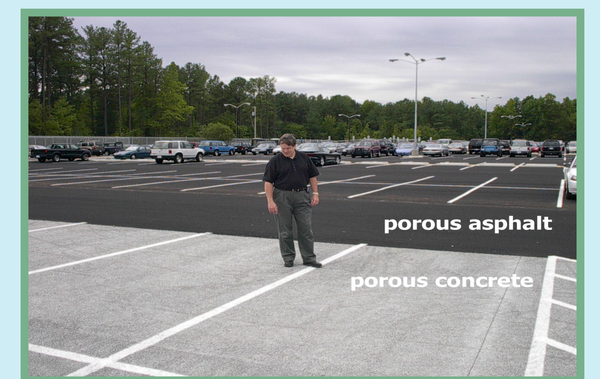
Porous Asphalt Parking Lot at the University of North Carolina at Chapel Hill, NC.
